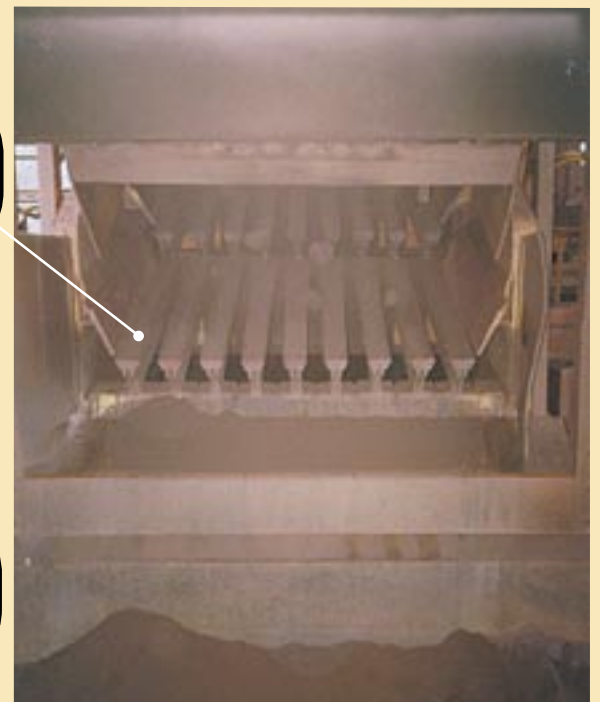
Custom wear plates stud bolted in an iron ore chute loader (left).
