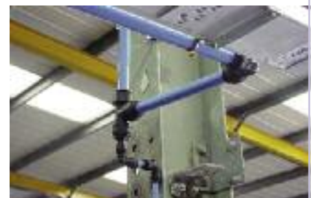
5. System complete in 2 days
